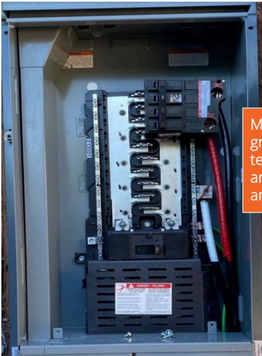
Photo: Meter/Main Service Panel (MSP) or Home Main Load Center
