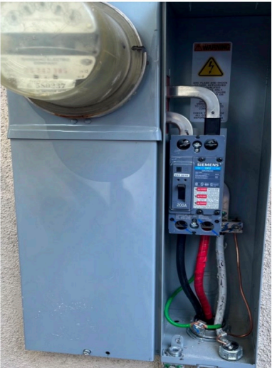
Photo: Meter/Main Service Panel (MSP) or Home Main Load Center
