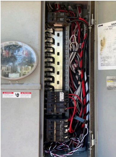
Photo: Meter/Main Service Panel (MSP) or Home Main Load Center
