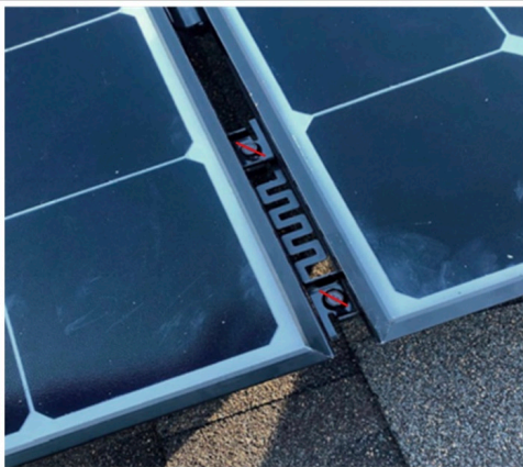
Sample photo confirming the use of torqued row-to-row grounding clips on-site.
